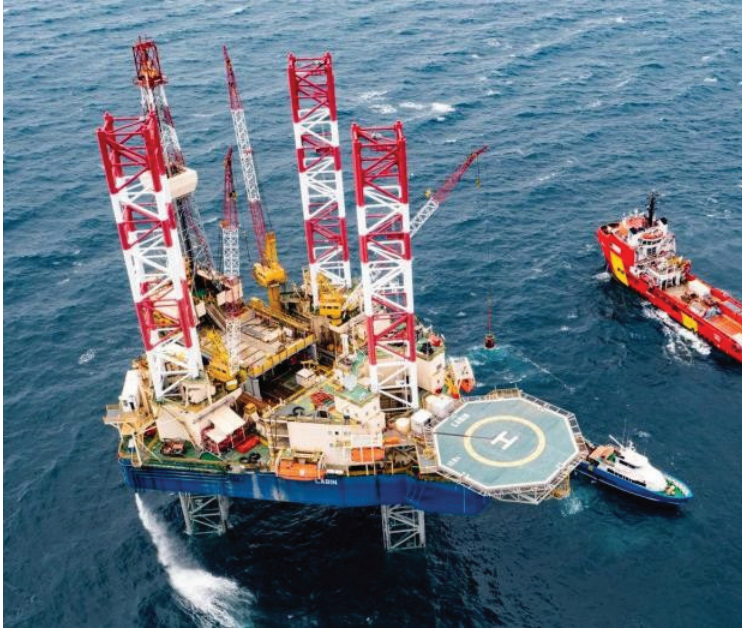
Figure 1: The Jack up oil platform
