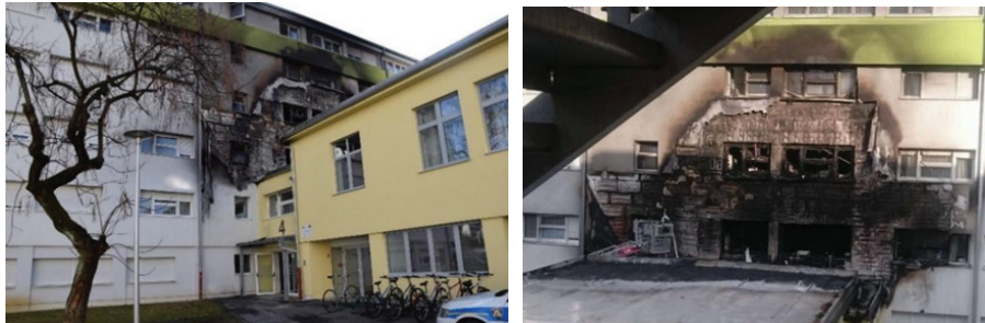
Figures 1 and 2: Fire and damage of front in student dormitory
