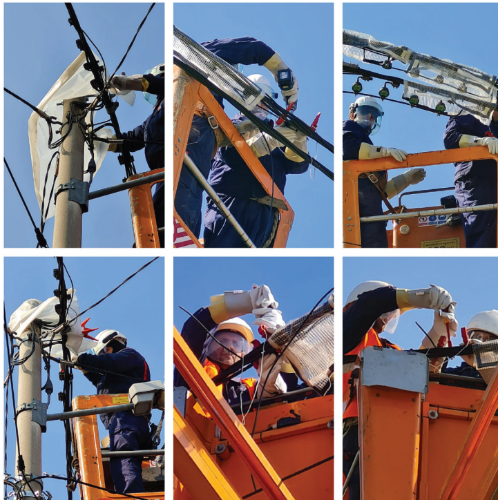
Figure 1: Live working on overhead lines 0.4 kV in Elektra Zagreb
